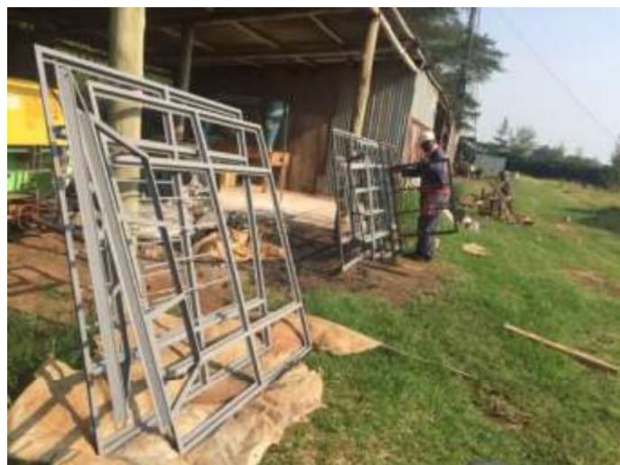
New windows being built on site
