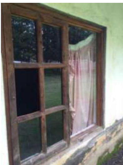
Old windows & outside wall
